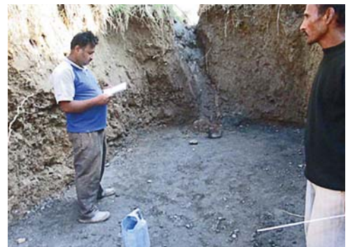
Work is starting on the first reed bed
